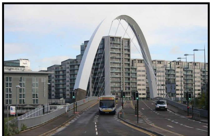
Two lanes of the "Squinty Bridge" are reserved for Fastlink buses. The bridge is designed to be capable of taking light rail vehicles at some time in the future.
