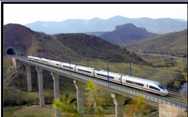
HS2 to Scotland will cross the Southern Uplands. A Siemens high speed train (above) is pictured in hilly country in Spain.
