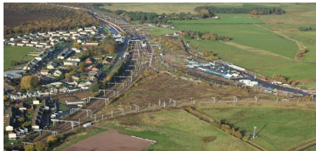
Carstairs Junction was completely rebuilt in 2023 by Network Rail. Photo: NR
