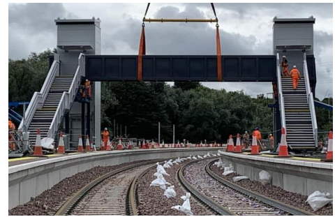
Photo of Cameron Bridge: Network Rail
