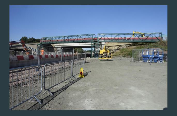
With the Bawbee Bridge reconstruction, a pipe bridge carried utilities over the line
