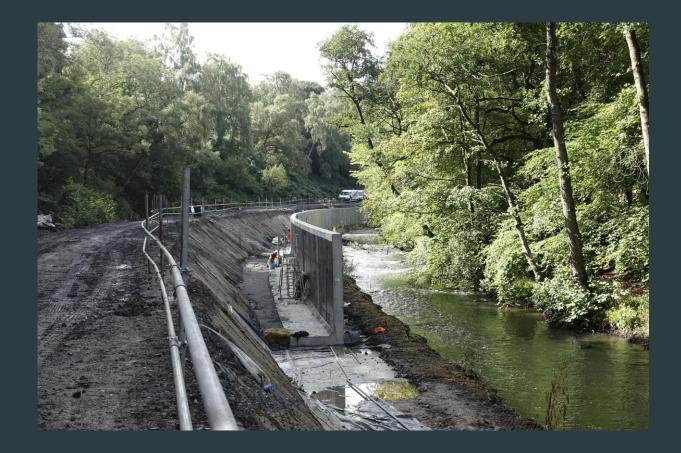
Further East at Cardowie, engineers constructed a flood protection wall by the Leven
