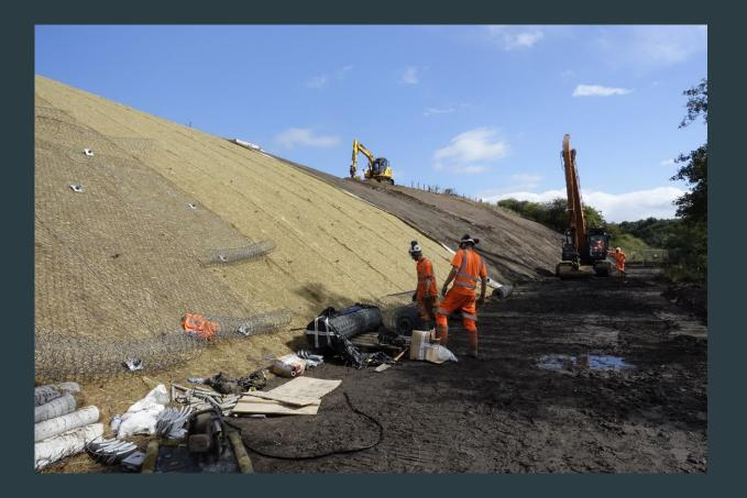
By June 2022, a 'green mat' to stabilise a slope was being installed at Tullybreck
