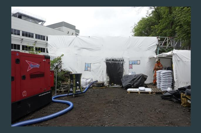
Restoring ten girder underbridges (as here at Cameron Bridge) required encapsulation
