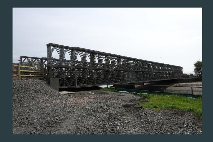
With the closure of the Bawbee Bridge, a large Bailey bridge was installed at Levenmouth
